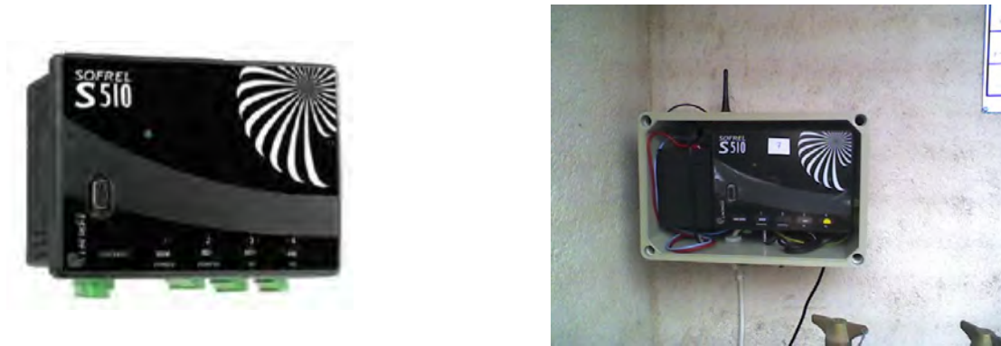
FIGURE 81. REMOTE CONTROL STATION. RIGHT (INSIDE THE PROTECTIVE BOX IP 68)
